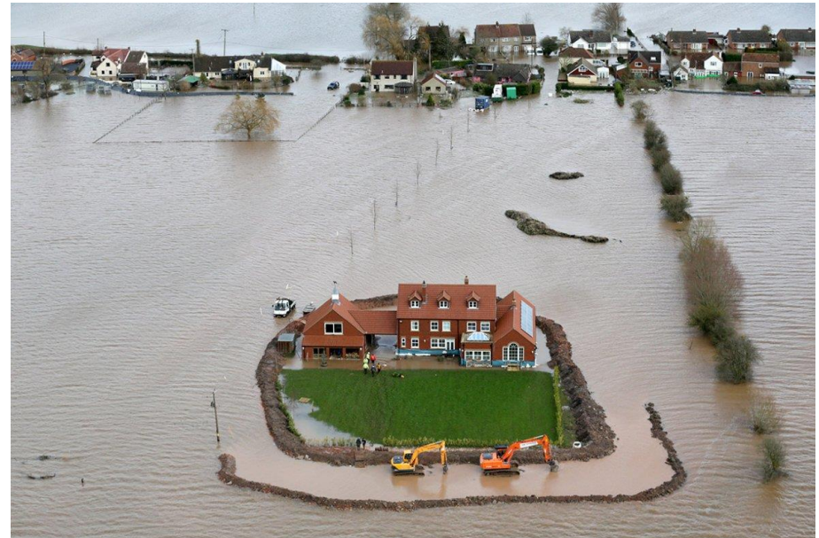
Flooding on Somerset levels 2014
